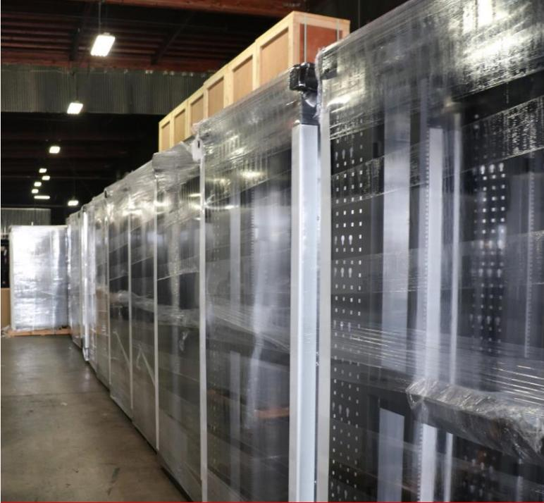
Many organizations are turning to off-site integration processes to minimize the disruption associated with installing, configuring and integrating equipment within the data center environment. System integrators “rack and stack” equipment in fully configured units and deliver these to the customer’s site.
